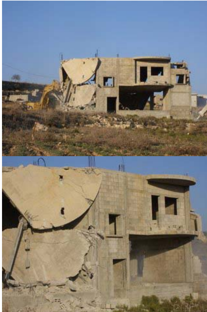
- Caterpillar & Volvo equipment demolishing house in Al Funduq, West Bank
