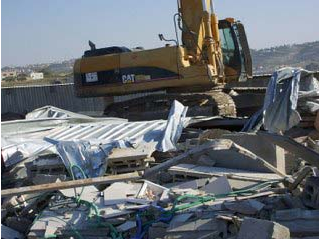
Agricultural Demolition, Al Funduq, 22nd nov '06 – CAT and Volvo shown
