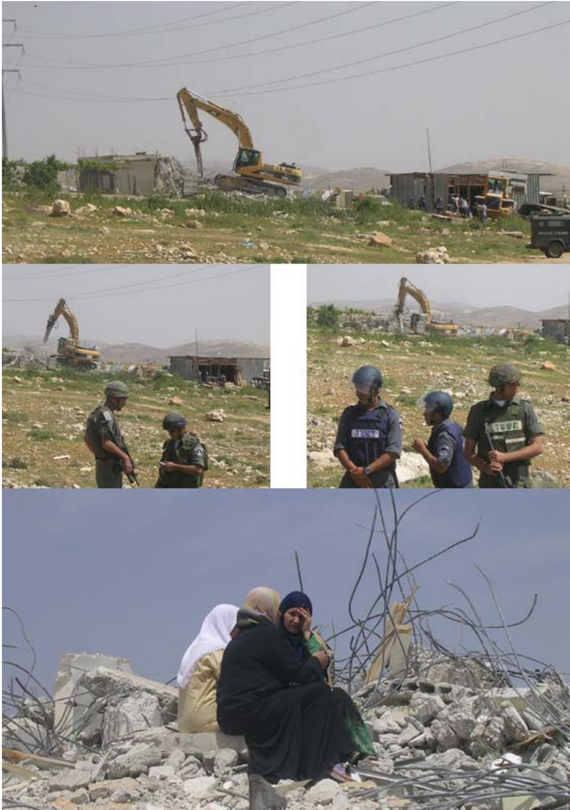
Caterpillar demolition of homes in Anata
